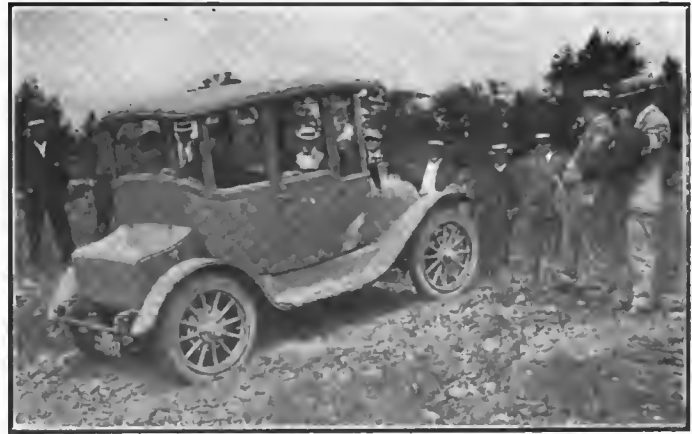
Demonstration of new Buffalo electric before automobile men and electrical engineers
